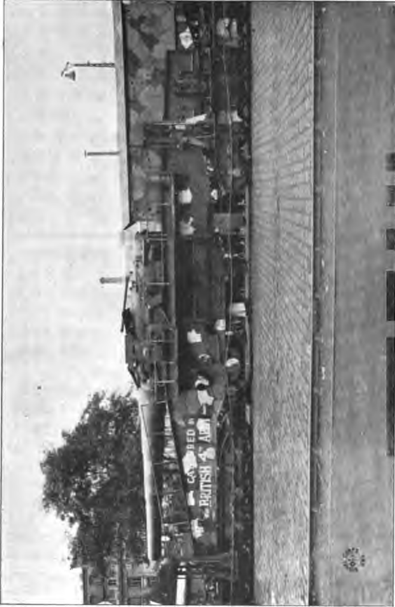
280-MM. GERMAN GUN ON RAILWAY MOUNT (LEFT SIDE).
